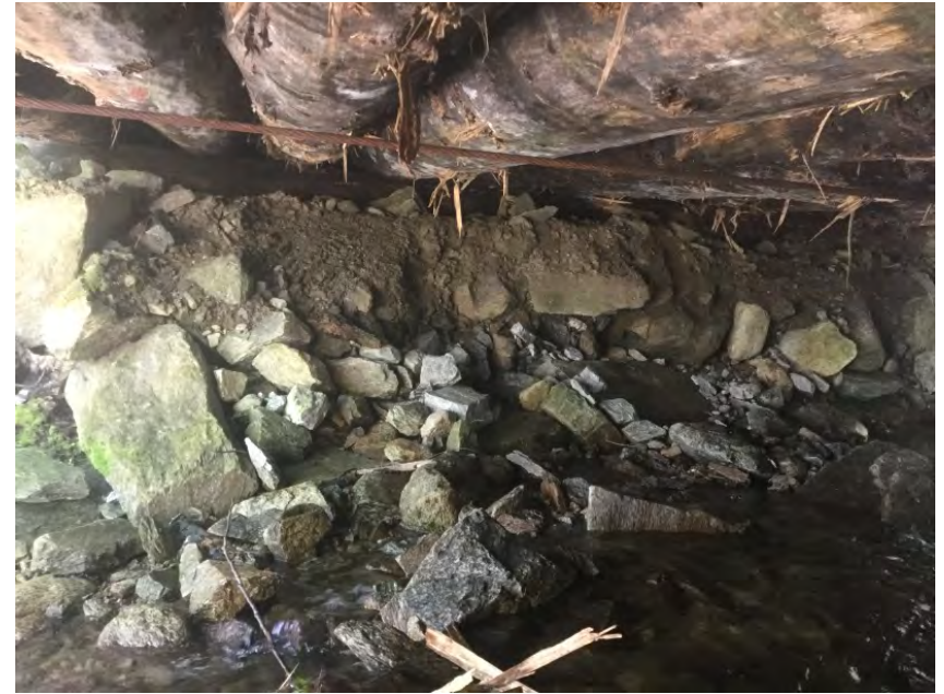
Right Bank Abutment when facing downstream
