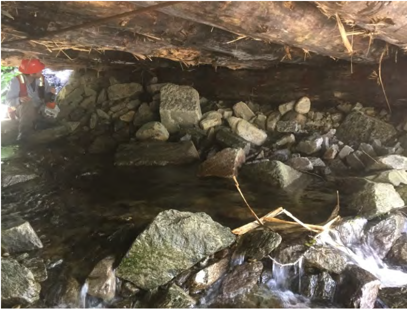
Left Bank Abutment when facing downstream
